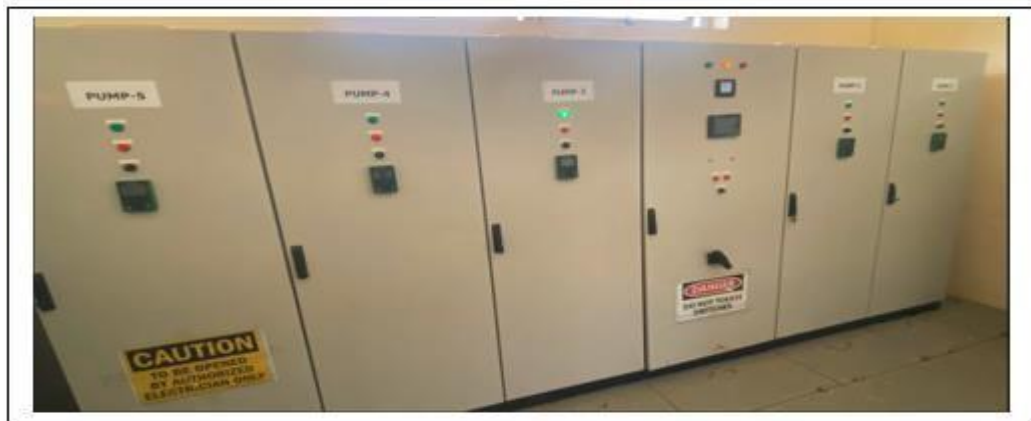
Fig. 4.4 Picture of the Five VFD at the Low-lift Section of the Plant
